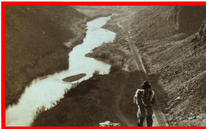
A Native American looks down at a newly-completed section of the transcontinental railroad. Nevada , about 1868
