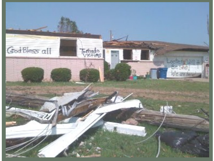
Joplin Tornado Damage
