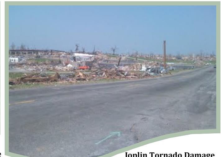
Joplin Tornado Damage
